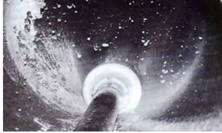
Cement lining grinding
